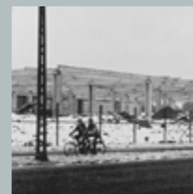
Bellahøj construction in 1965
